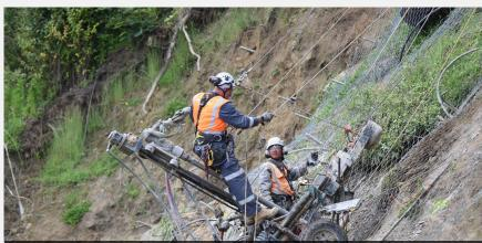
Regular maintenance work and remedial work on slip sites like this high, destabilised slope near Parnell Tunnel will continue. This slip started on Auckland Anniversary Weekend when vast amounts of water followed a natural flow path from the area around Auckland Museum. Permanent repairs include putting numerous rock anchors into the bedrock to stabilise the layer of loose rock.
